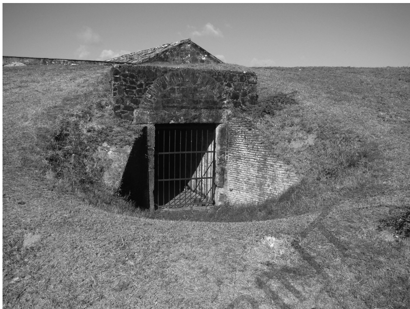
Figure 10.5. The waterfront gate of Fort Margaretha, Paraíba (1634), constructed of small Dutch yellow bricks. Photo by O. F. Hefting.
