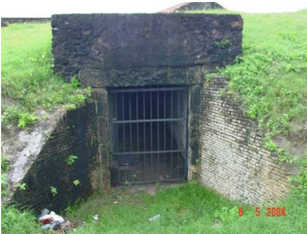
Picture 10. Dutch gate, constructed of Dutch yellow bricks, Fortaleza de Santa Catarina, Cabedelo, Brazil
